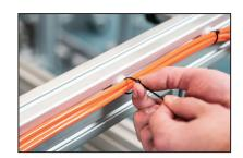
3. Insert cable tie to secure wire or cable run.
