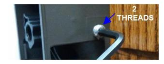
Make a note of the orientation of the cam. The opening of the cam should be directed toward the landing door. It is important that you install the new metal cam in the correct orientation.
