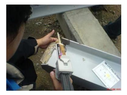
*Figure 4: handheld*  $3M^{TM}$  *EPX Plus II applicator containing a duo-pak cartridge with attached static mix nozzle.*
