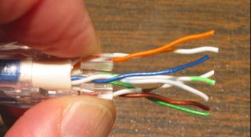
Untwist the wire pairs. Stop untwisting at the edge of the wire aligner.
