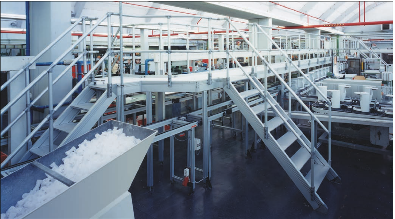
Crossovers made from ITAS elements provide access to various production areas.
